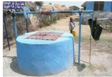
Use only covered wells
